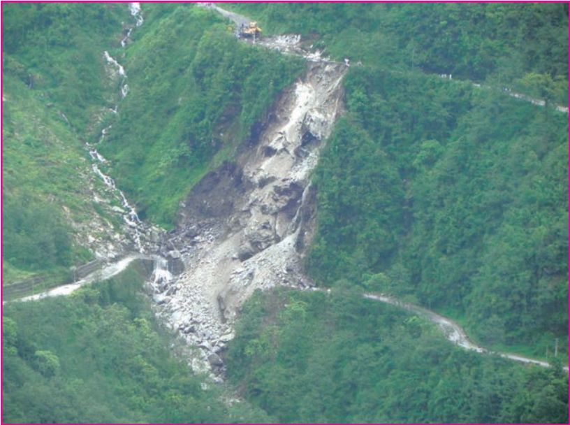
Landslide affecting roads, buildings, vegetation and drainage system
