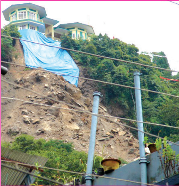
Landslide poses threat to the safety of buildings
